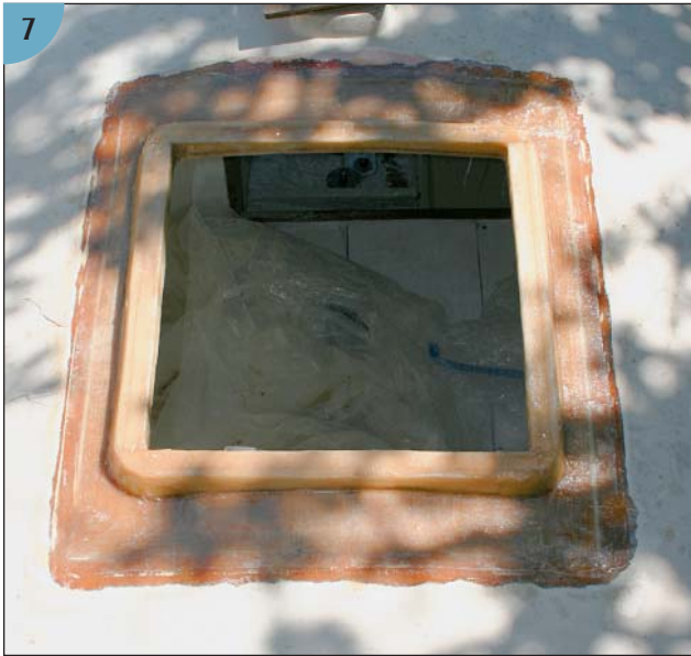
(7) We then laid up two layers of 6-ounce cloth over the exterior joint, up over the boss, and down through the hatch opening and over the deck underside to lap the existing inner skin, into which we had ground a scarf. When the fiberglass had set up we sanded the entire area smooth and faired it into the surrounding deck. This shows the laminate before it was coated with fairing and sanded smooth.
