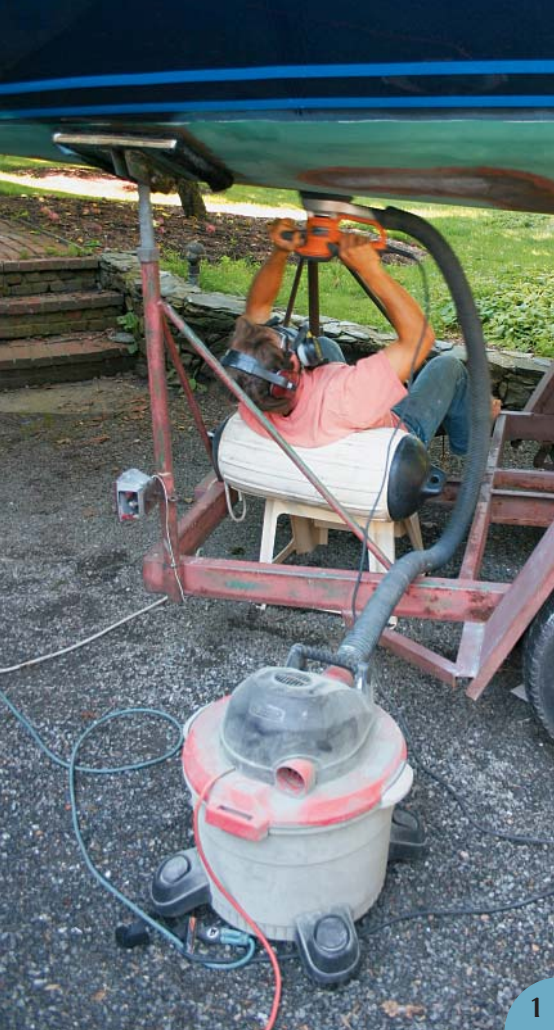
(1) My RIDGID 6-inch random orbit sander attached to the RIDGID shop vac. This method may look a little ungainly, but it keeps the job free of sanding dust and residues. You do, however, need to make sure the holes in the sanding disks align with the holes in the sanding pad. (2) Notice how little dust is generated around the sander in use. Even so, the operator is wearing a respirator and eye and ear protection.
