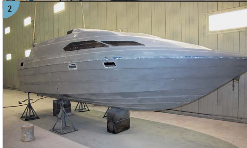
(1) Sanding a primed hull and deck to prepare them for the topcoat. (2) A boat primed and ready for a topcoat.
