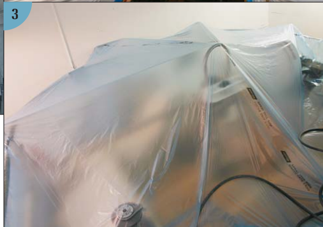
(1, 2, 3) The fiberglass on this boat will be ground back, which will spread fiberglass dust everywhere. To avoid removing all the interior fittings and cushions and having to painstakingly clean the boat after the repair work is done, the workers have taped polyethylene sheeting over all areas not involved in the repair.
