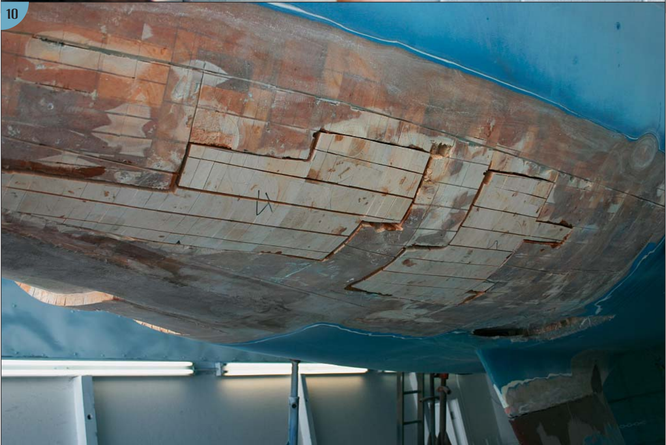
(9) Then they pressed the new core into place and clamped it until the resin hardened. (10) The finished core patch.
