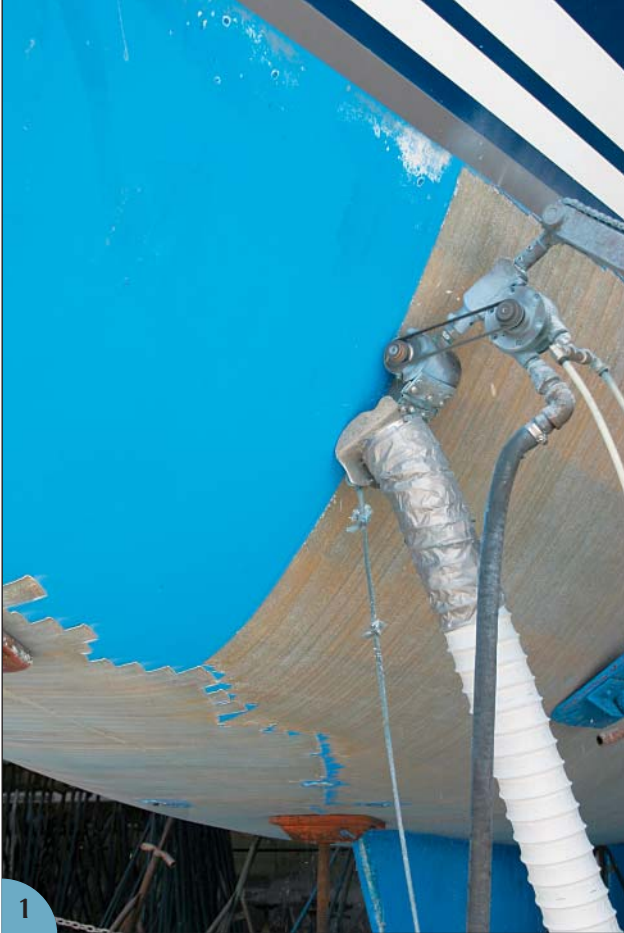
(1) A peeling machine at work in the Jamestown (Rhode Island) Boat Yard. This machine has a small rotary planing head about 3 inches (75 mm) across. It can be set to a pre-determined depth, and as it moves down the hull, it peels away both the gelcoat and the underlying layer of CSM. If the hull has a core that has been penetrated with moisture, a second peel is usually done to remove the entire outer laminate.
