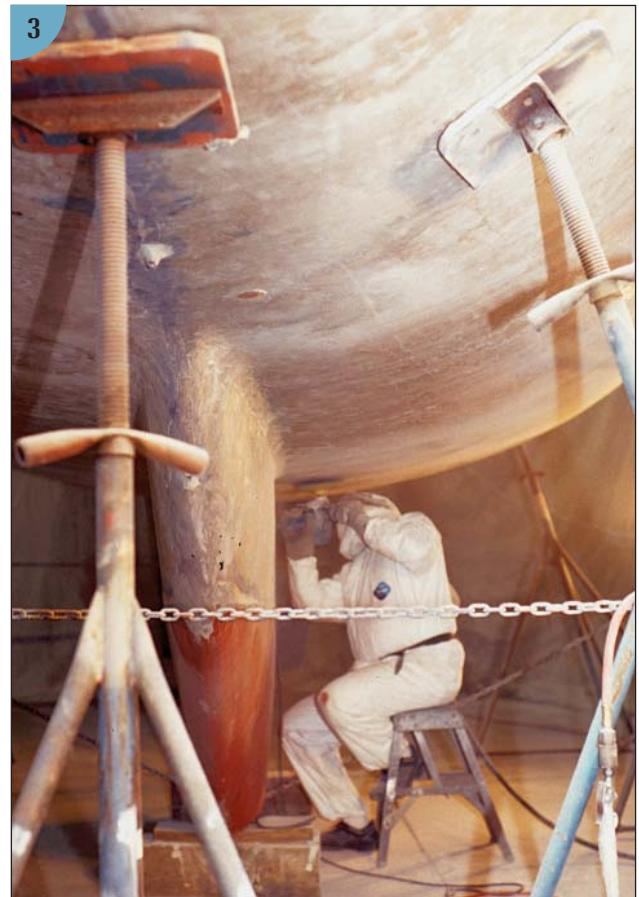
(3) After a hull has been peeled, a worker finishes the job by grinding off areas the peeler head can't reach.
